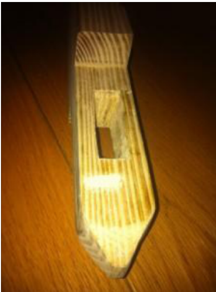
Mortise in the end of a stretcher
