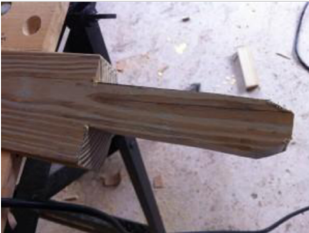
Cutting the ends of the stretchers
